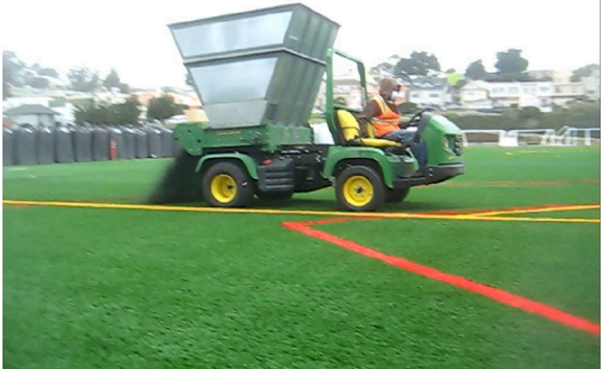
Figure 3.2 Semi-mechanised application of infill
