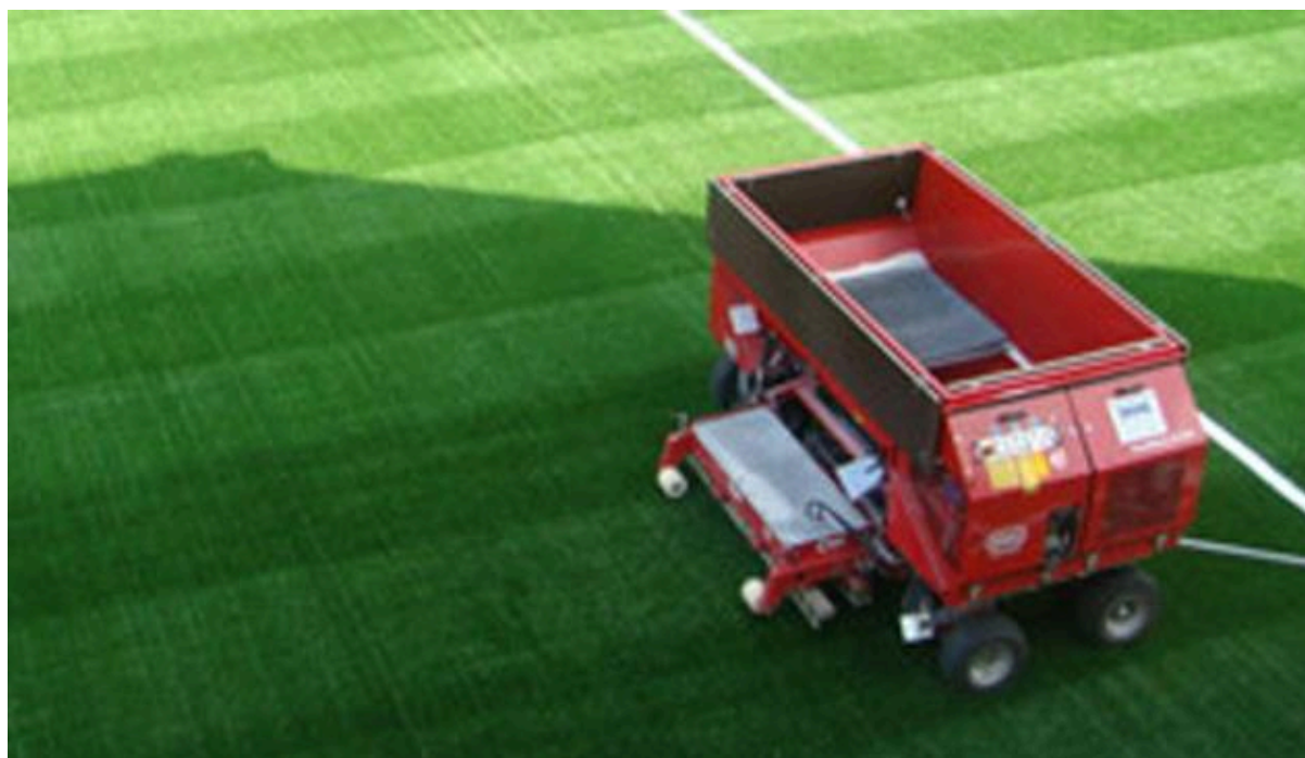
Figure 3.1 Mechanised application of infill (photo submitted by ESTO)
